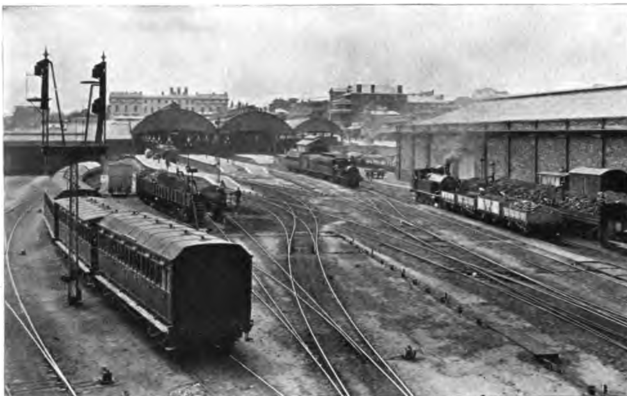
VIEW OF ADELAIDE RAILWAY STATION FROM MORPHETT STREET BRIDGE.
